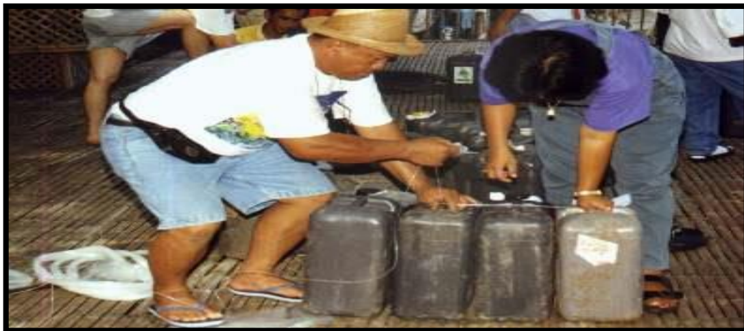
Figure 23: Making floating raft with plastic container
