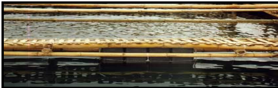
Figure 22: Attaching plastic containers to raft
