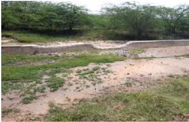
Hydrological problems in Varavani Tank Weir Partially Broken: Water is not stored to its full capacity. Hence the quantity of water supplied to irrigation is getting reduced. Rectification to this work is of minor in nature and should be carried out immediately.
