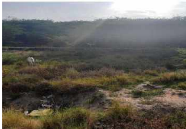
Hydrological problem- Kaikudi tank surplus with lot of vegetation obstructing the flow to Sholandur big tank and Encroachment need to be evicted.
