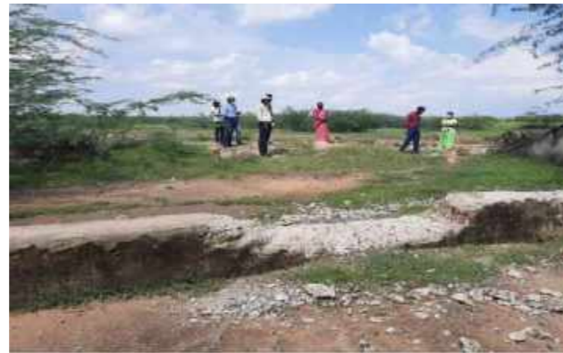
Hydrological problem is no defined course in weir of Varavani tank: Surplus water going through field. Action to be initiated for forming a course for the smooth and efficient flow of water to the lower tank.
