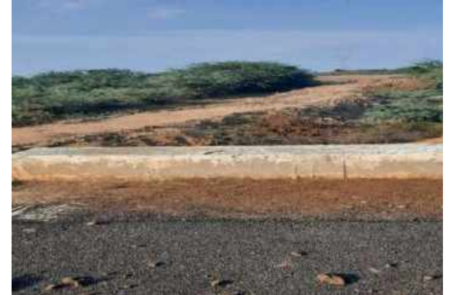
Hydrological problem- Illegal earthen bund across Peeyar river feeding Sholandur big tank which obstructing the natural flow. Rectification measures needs to be taken.
