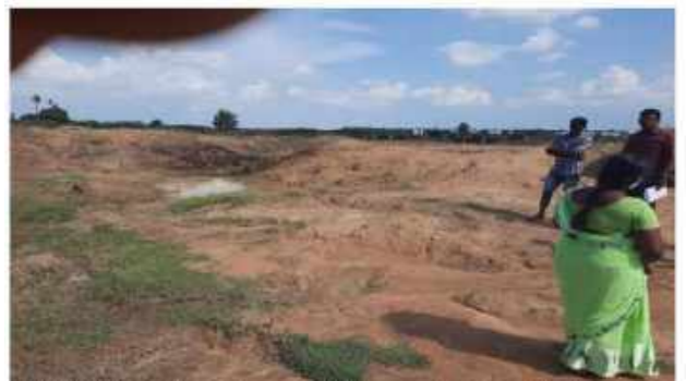
Hydrological problem- Water does not enter into the tank due to silting up of inflow point through Sarukaniar anicut to Kottakarai river. Necessary landscaping and allied works should be carried out to overcome this problem so that inflow to R.S.Mangalam tank is to be realized without any obstructions.
